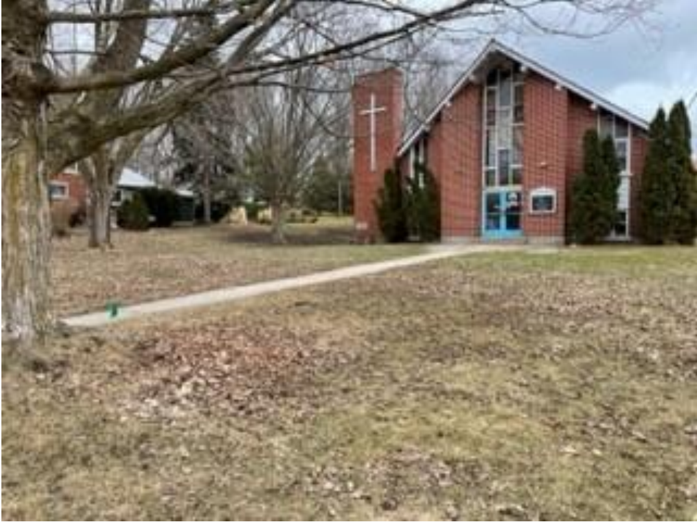
Figure 4 Existing Conditions – 175 Oxford Street
