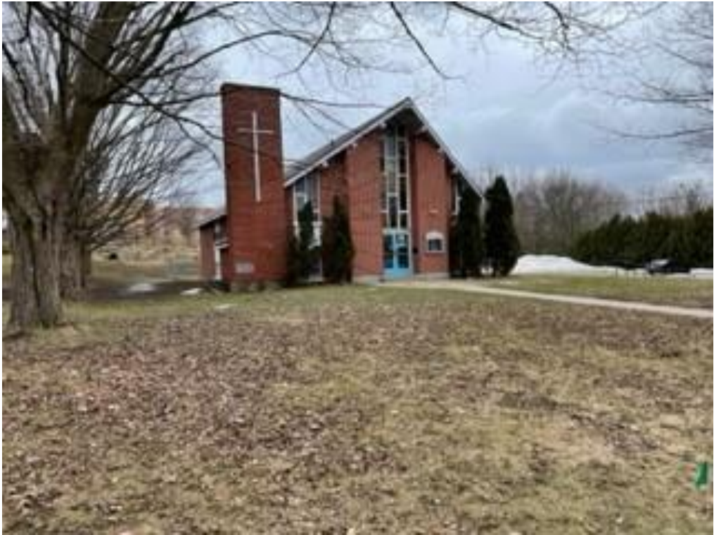
Figure 3 Existing Conditions – 175 Oxford Street (showing tree line along east property line)
