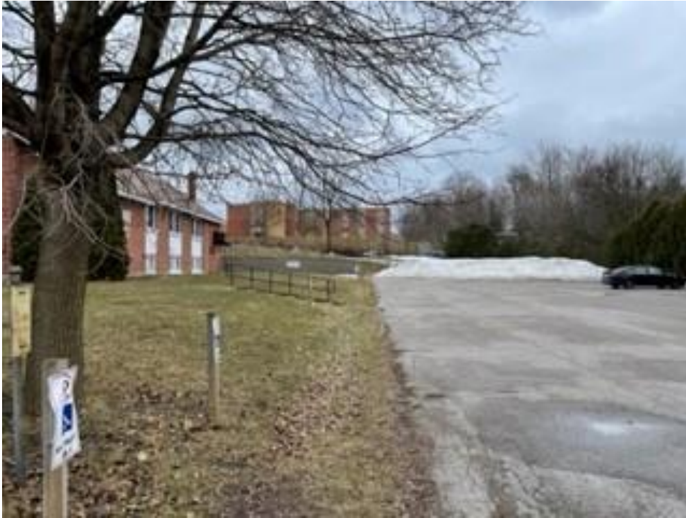
Figure 5 Existing Conditions – 175 Oxford Street (West side of property with Regent Park Public School in background)
