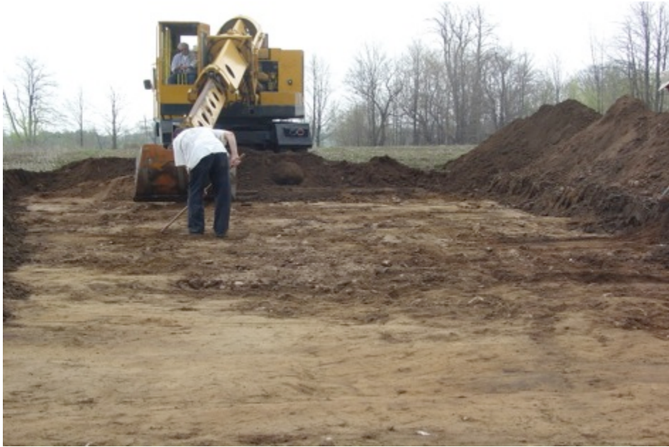
Plate 1 Topsoil Stripping of the Alia Kendra Site (BdGu-19)
