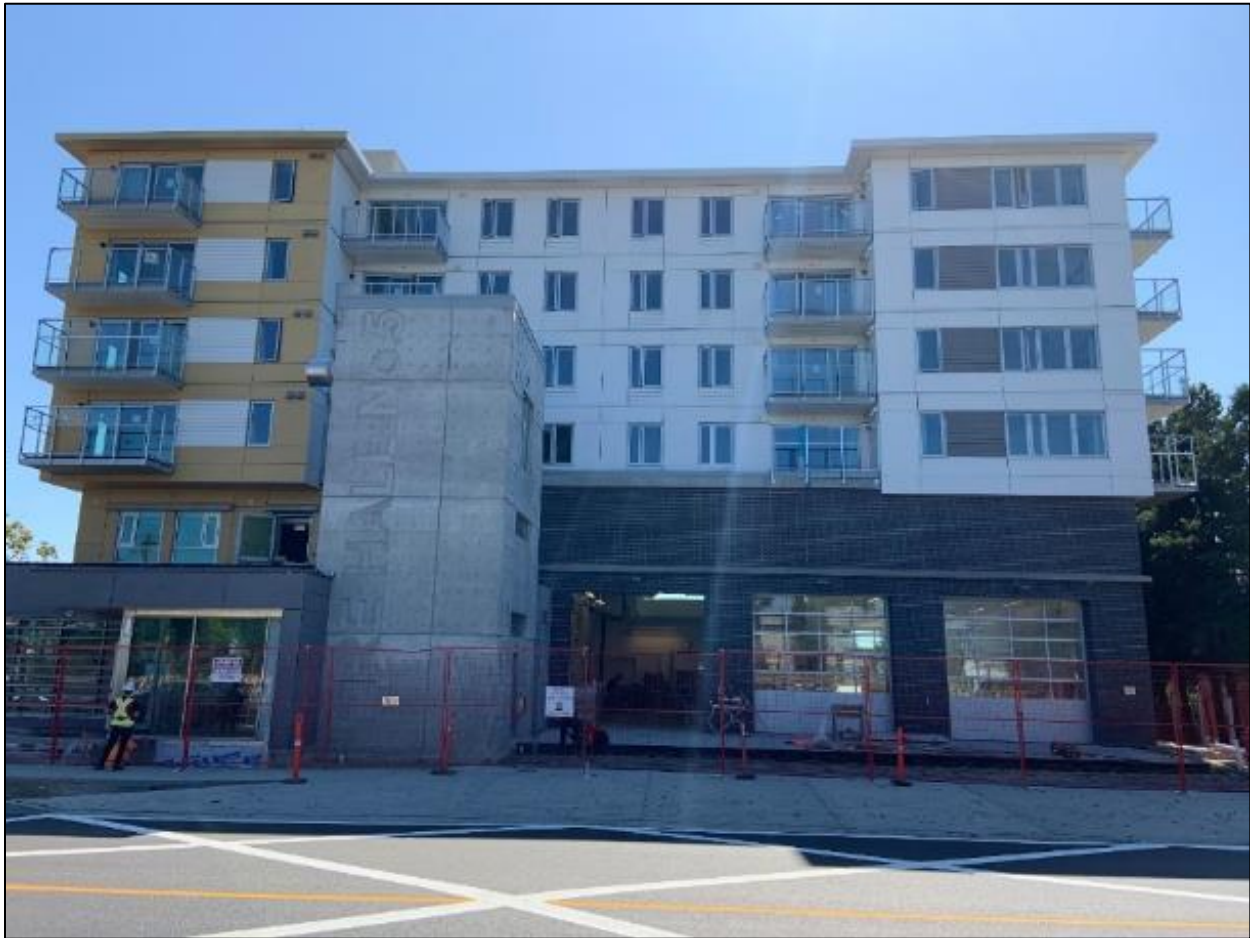
Figure 3 – City of Vancouver Fire Station #5
