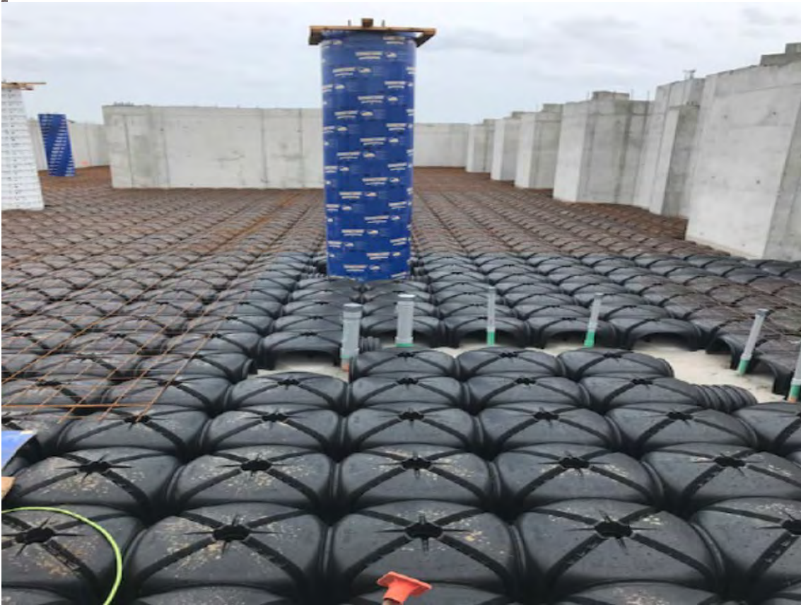
Cupolex Installation under Pool Change Rooms
