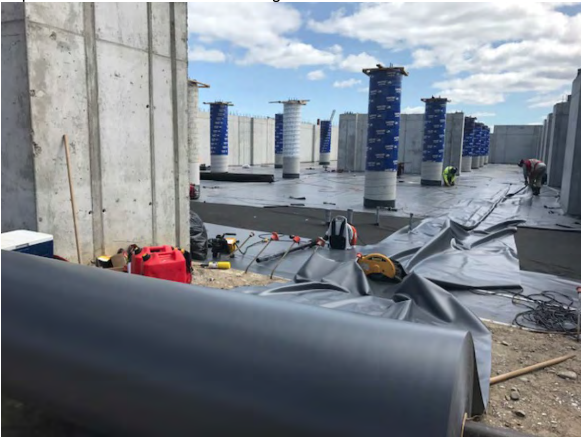
Gas Membrane installation over Cupolex
