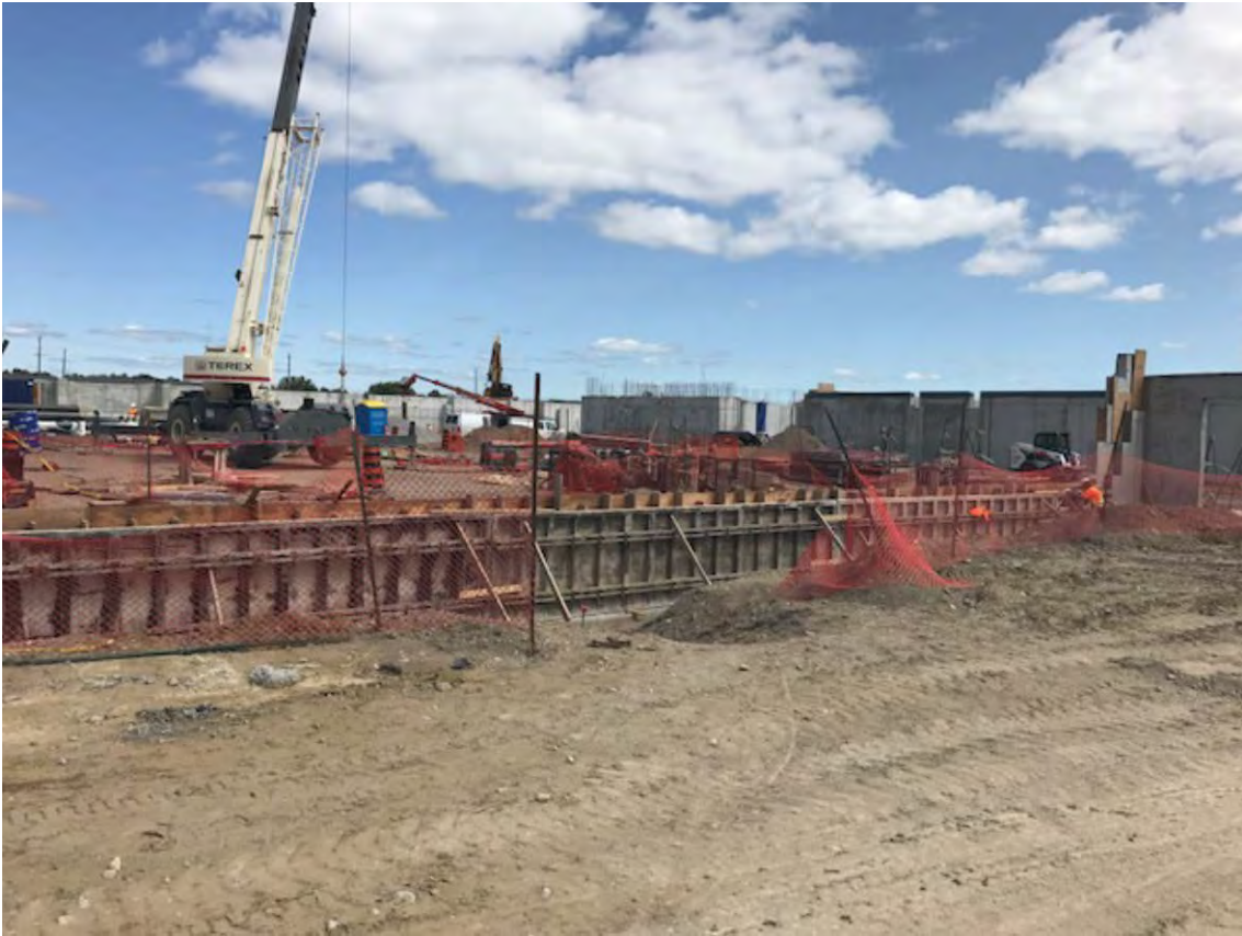
Building view to the south east
