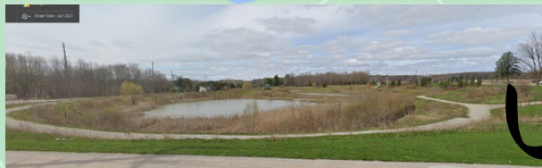
Site 4 - Stormwater Pond
