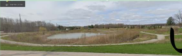
Site 4 - Stormwater Pond
