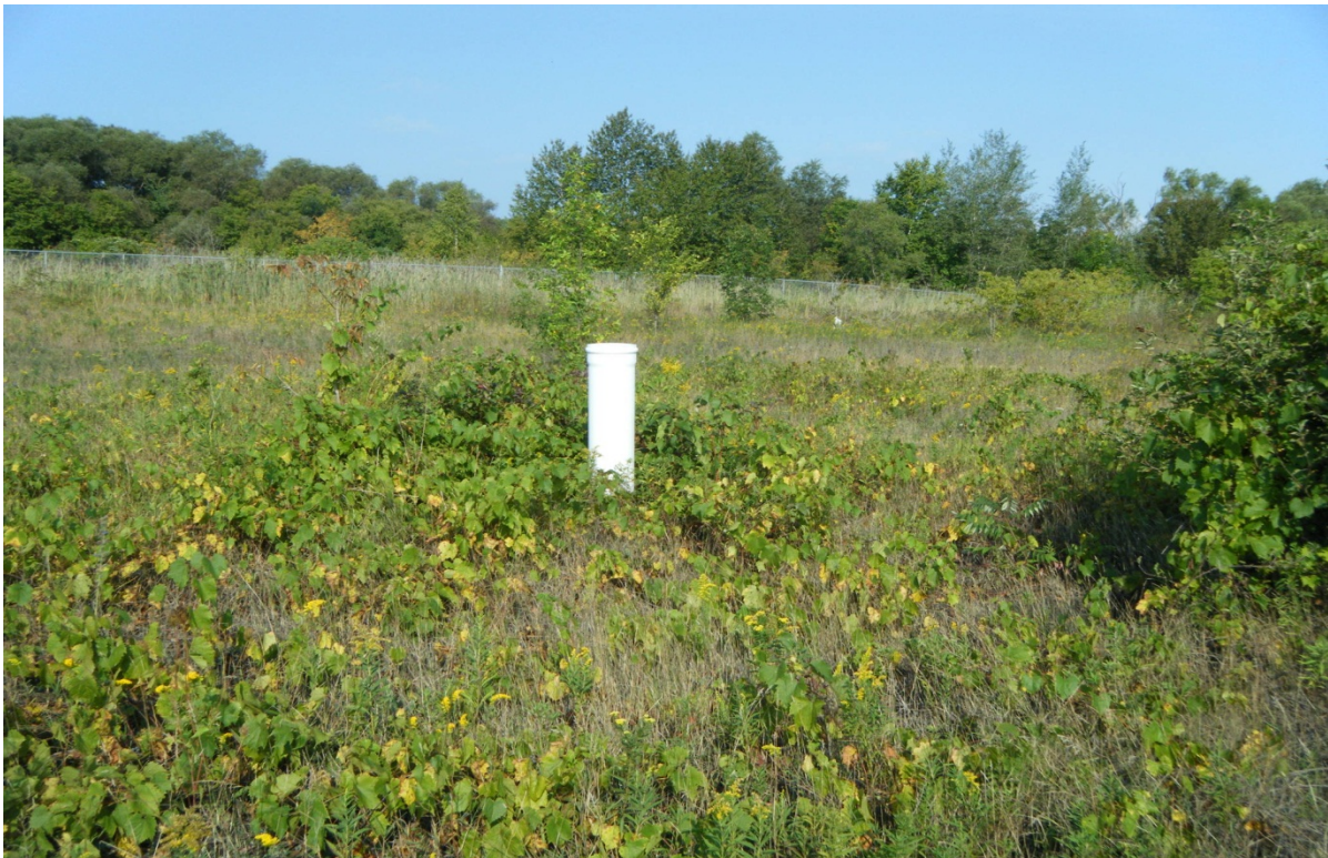
Photograph 4: View of sump or gas vent located in the Fill area at X4129
