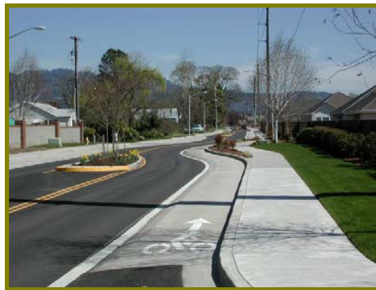
Figure 5.8 - Example of a Raised Bicycle Lane on Ayres Road in Eugene, Oregon 19
