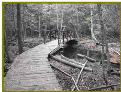
Figure 5.13 – Low Profile Boardwalk, Guelph, ON
