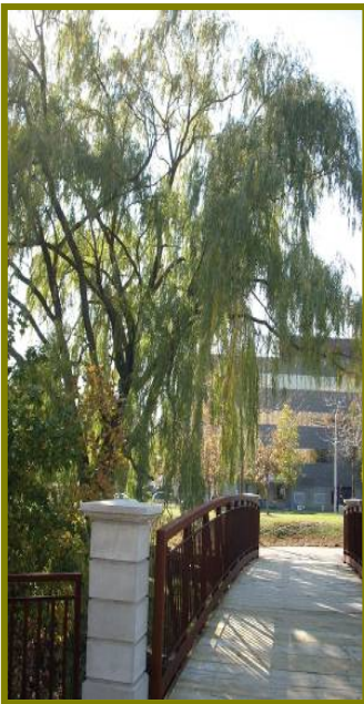
Figure 5.10 - A Pedestrian Trail Bridge, Brampton ON
