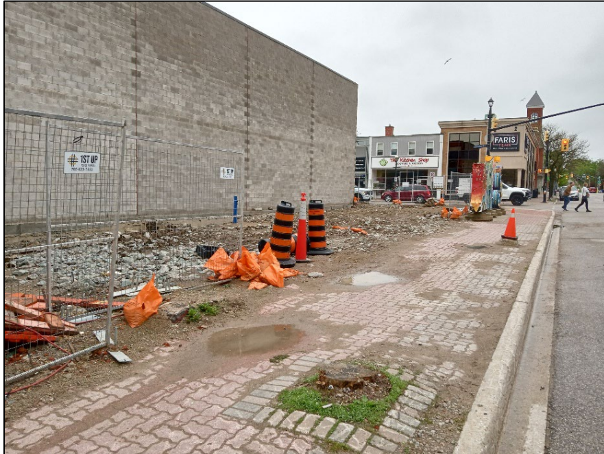
Figure 2 – Site Photo, May 24, 2026 (Staff)
