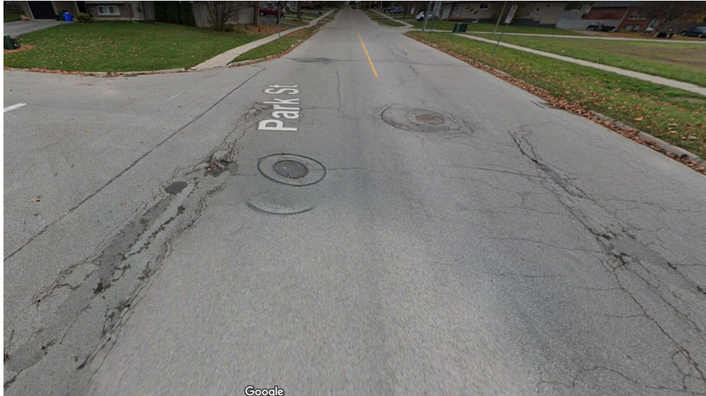
Park Street (Fittons Road West to Jordan Crescent) – PCI 55
