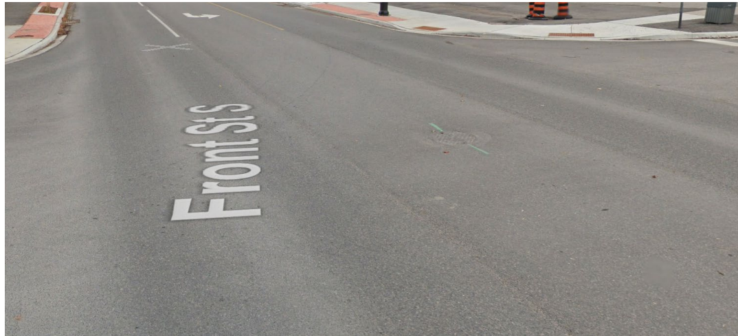
Front Street South – PCI 100
