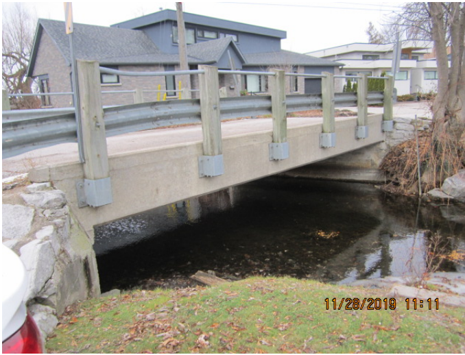
Cedar Island Bridge
