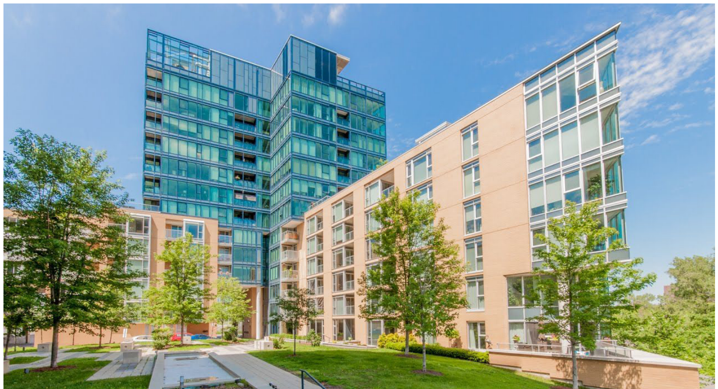
Figure 45. South Downtown is an appropriate location for taller buildings given the limited existing context.
