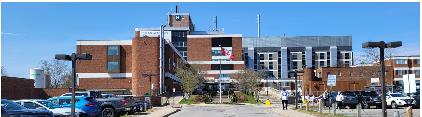
Figure 32. Institutions like OSMH bring vitality to the Downtown and attract other organizations and businesses. The site should continue to provide health care services while also accommodating commercial and residential uses.
