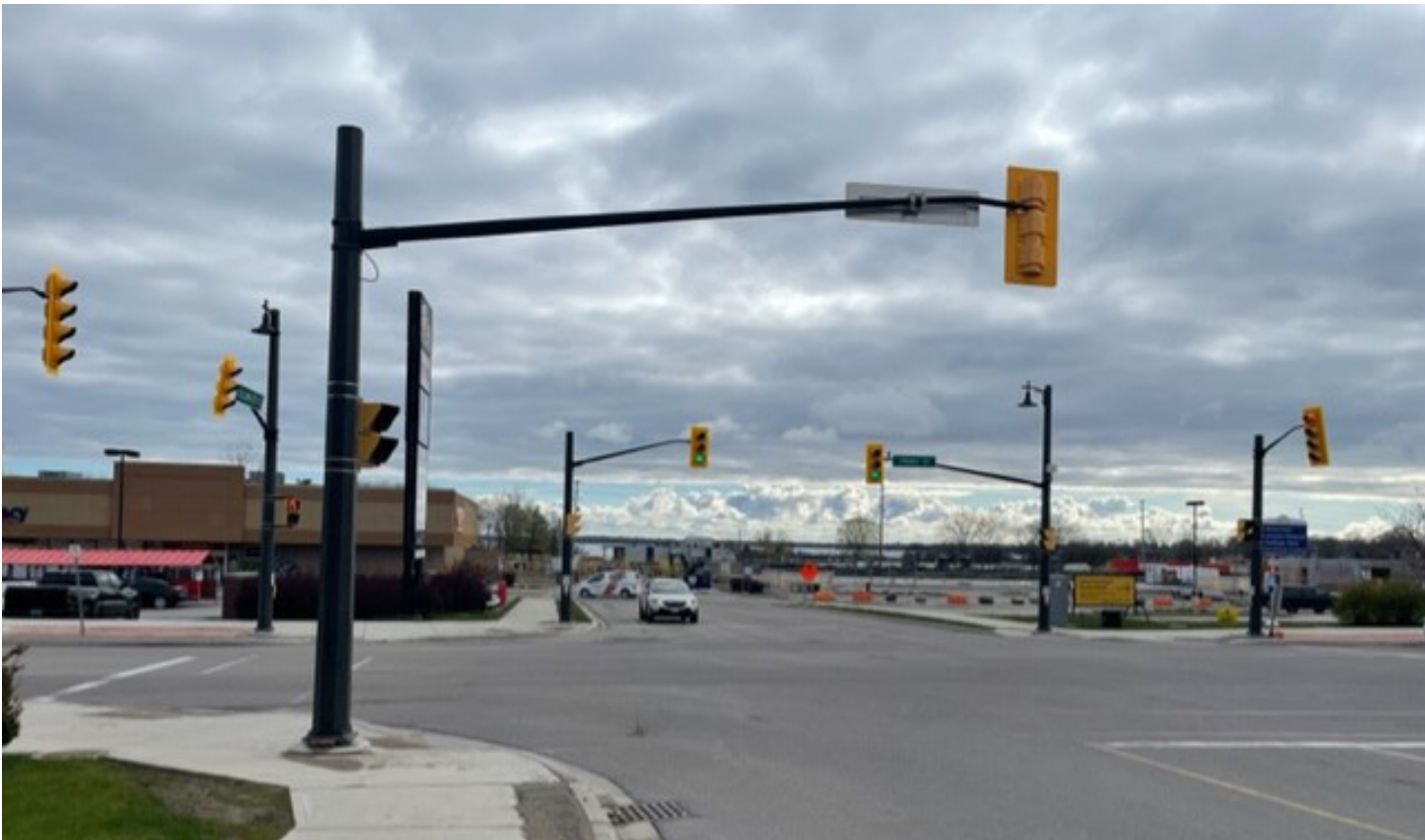
Figure 8. The extension of Coldwater Road to Lightfoot Drive established a new connection between Orillia's historic Downtown and its waterfront. Upgrades to below-grade municipal infrastructure sets the stage for new development.
