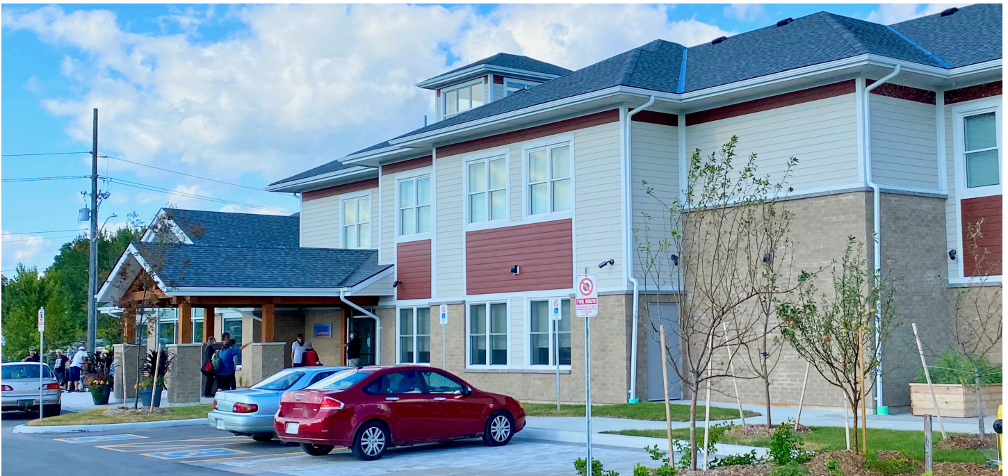
Figure 3. Lighthouse Community Services & Supportive Housing provides vital services to the County's most vulnerable populations. Like other community across Canada, Orillia is experiencing an affordability crisis and a growing homeless population. Source: Orillia News
