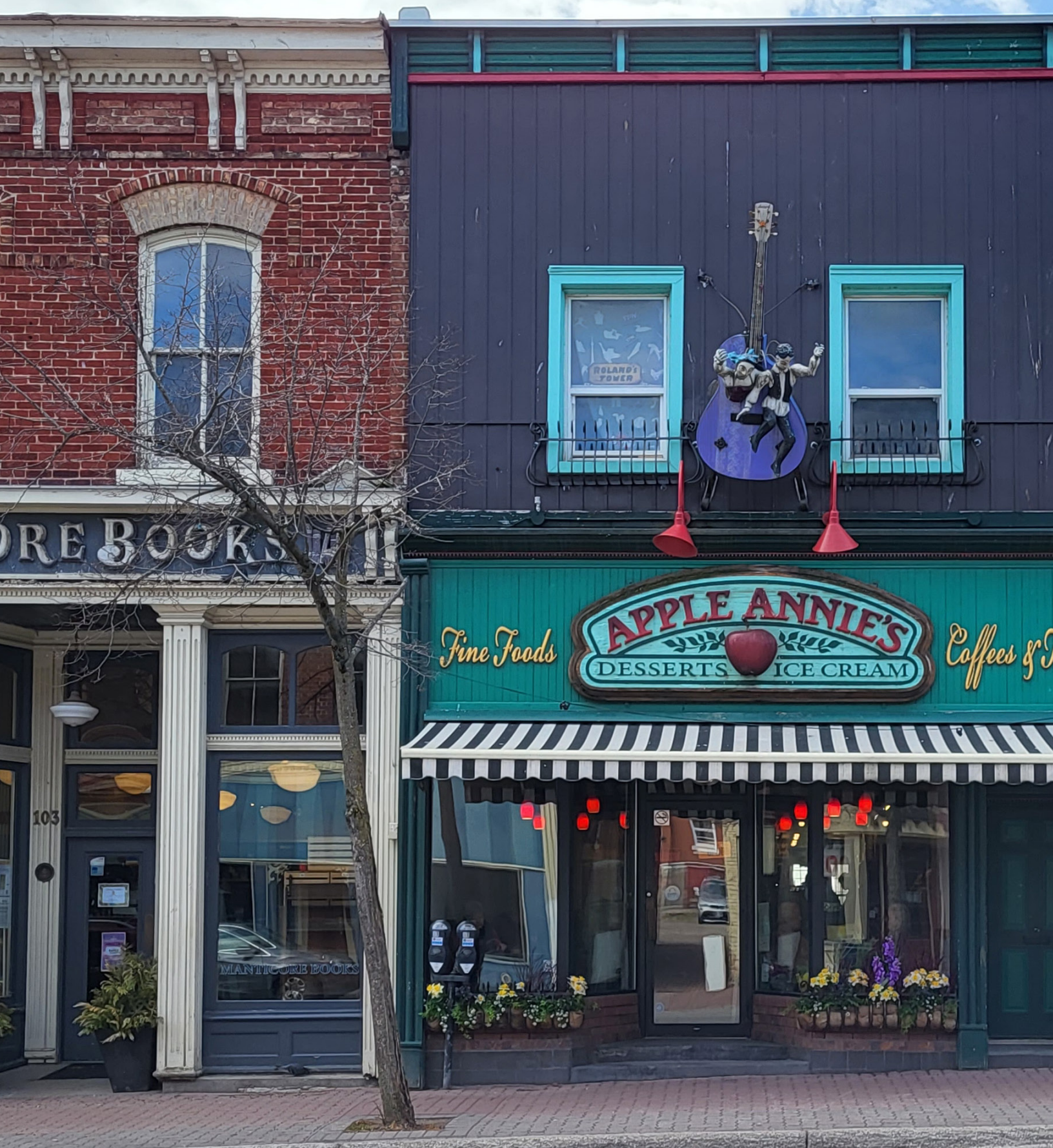
Figure 20. Apple Annie's received grant funding through the Downtown Tomorrow Community Improvement Plan. The business's expansion included a new accessible entrance at the rear of this Mississauga Street building.
