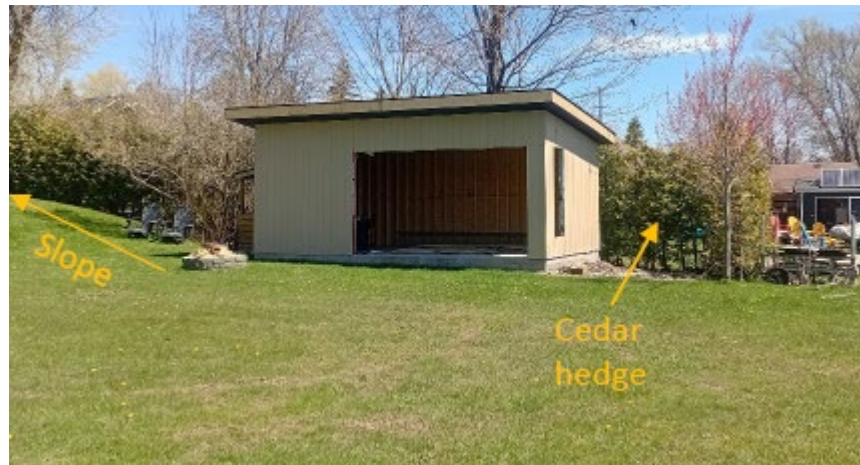
Figure 3 – View of Existing Structure
