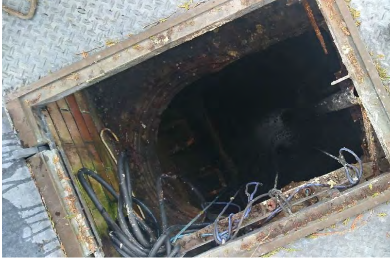
Figure 4 – Pumping Station No. 3 Wet Well
