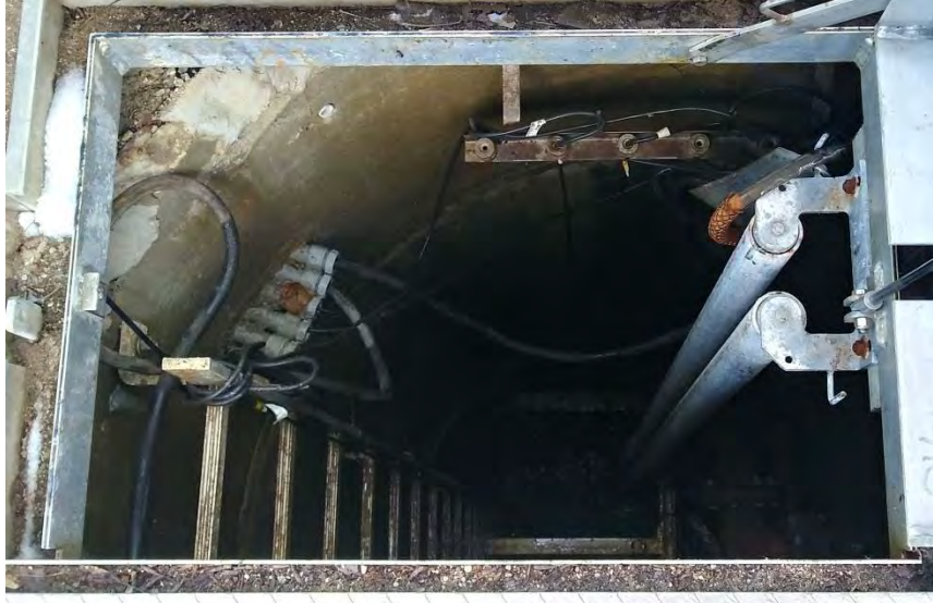
Figure 14 – Pumping Station No. 11 Wet Well
