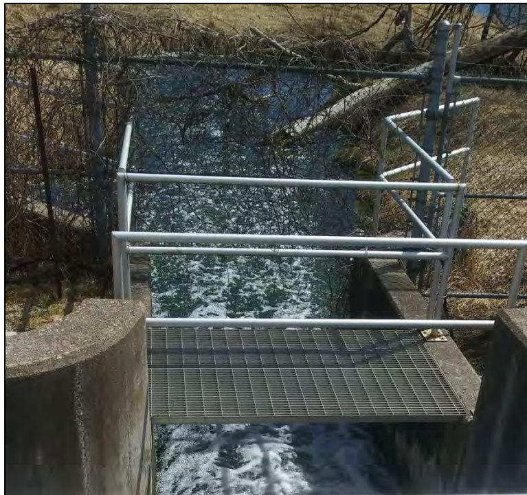
Figure 12 – Orillia WWTC Outfall
