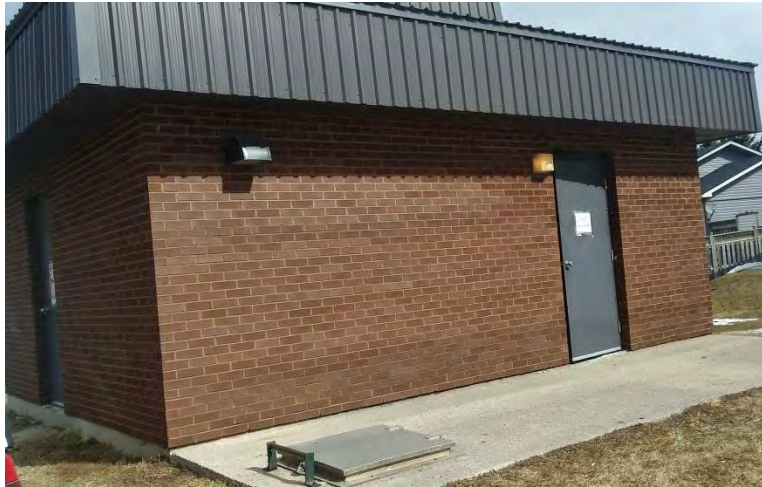
Figure 23 – Pumping Station No. 18
