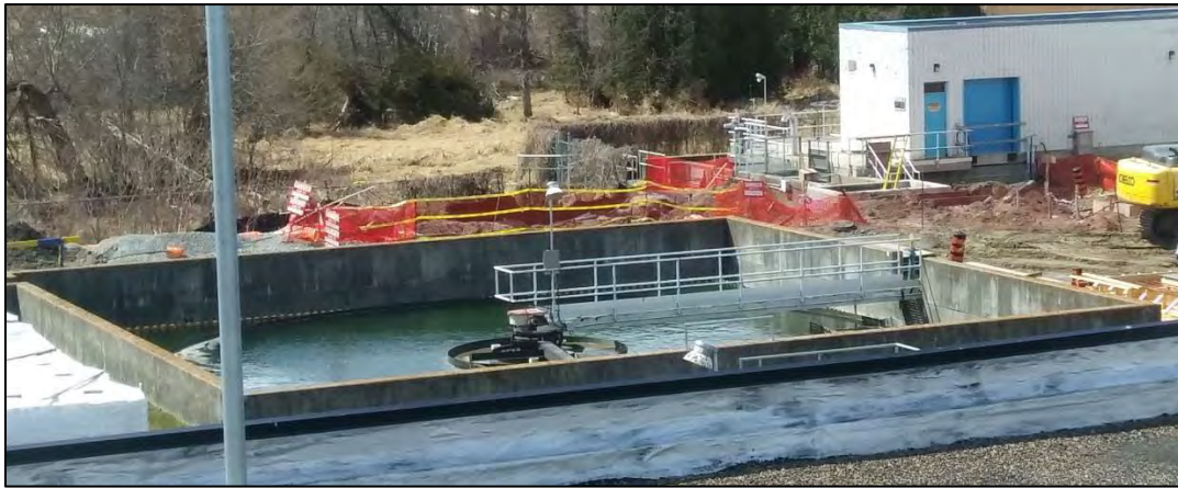
Figure 6 – Secondary Clarifier
