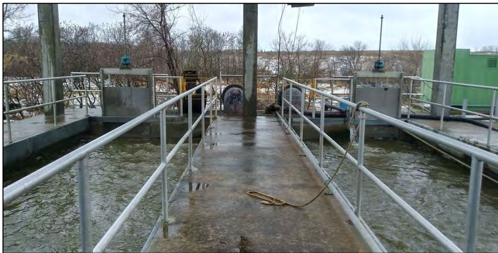
Figure 3 – Intake Grit Chamber
