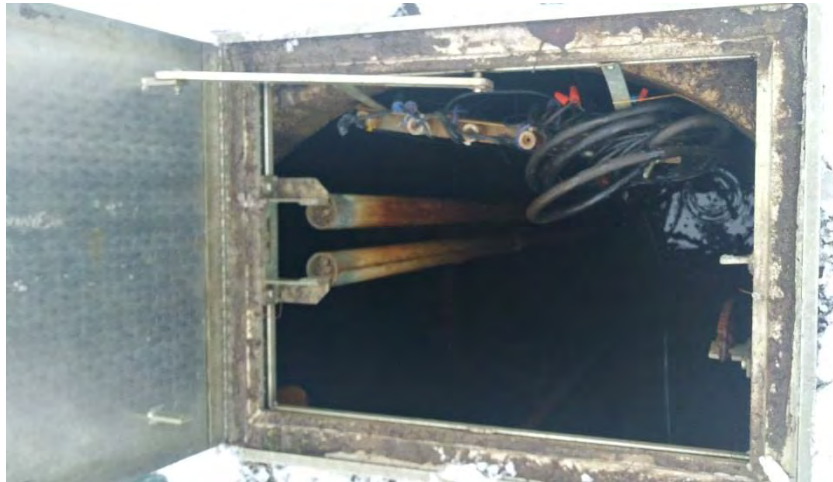
Figure 9 – Pumping Station No. 8 Wet Well
