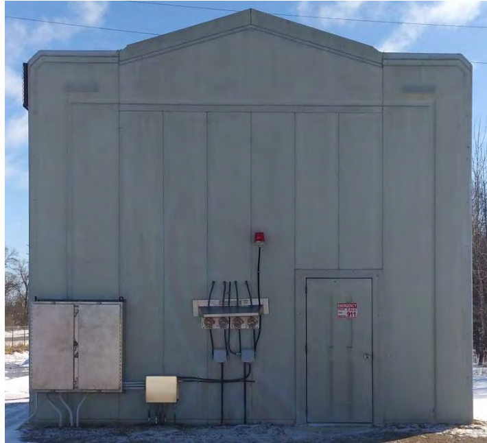
Figure 1 – Septage Receiving Station
