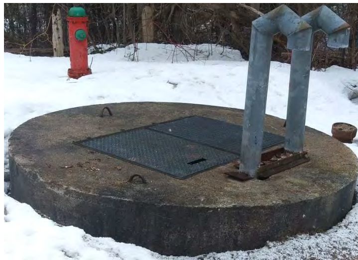
Figure 29 – Pumping Station No. 22
