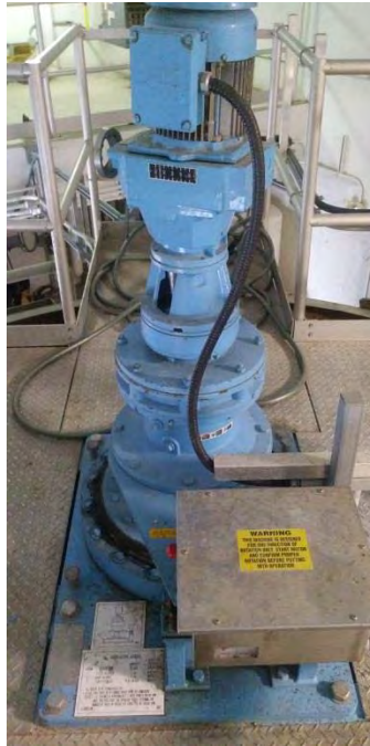
Figure 7 – DAF Rotor Motor
