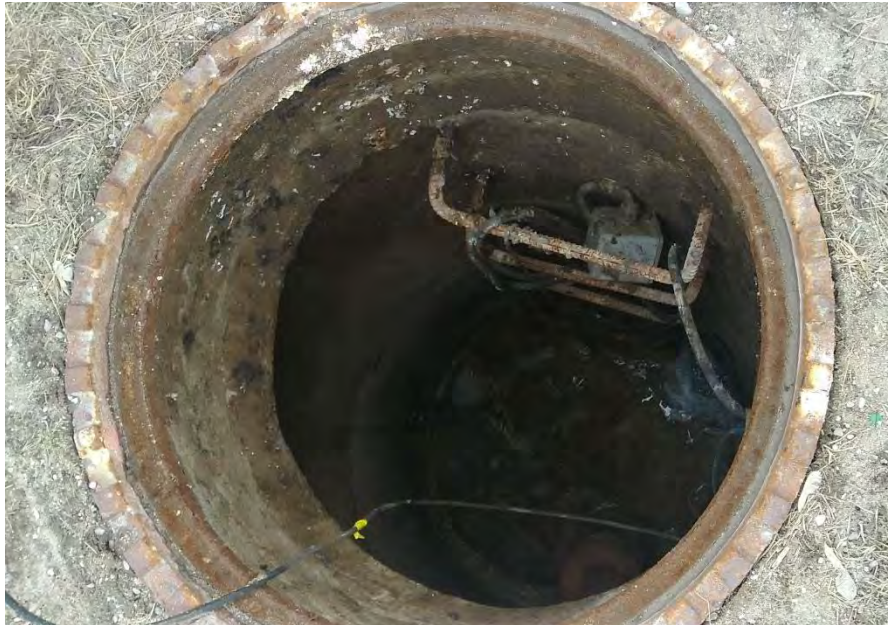
Figure 8 – Pumping Station No. 7 Wet Well
