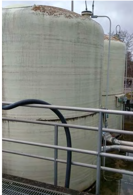
Figure 9 – Alum Tanks
