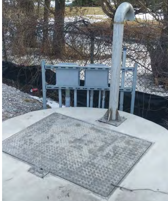
Figure 10 – Pumping Station No. 9 Wet Well
