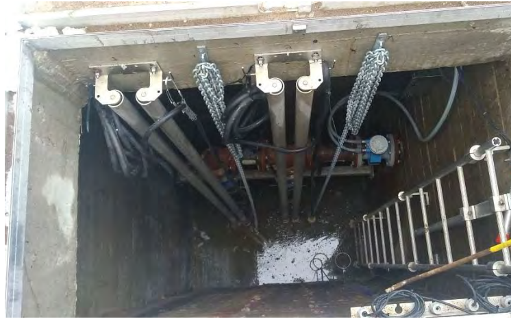
Figure 19 – Pumping Station No. 14 Wet Well
