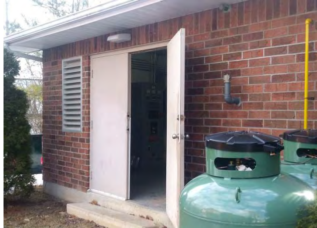
Figure 32 – Pumping Station No. 24
