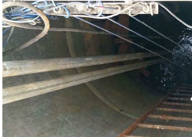
Figure 22 – Pumping Station No. 17 Wet Well
