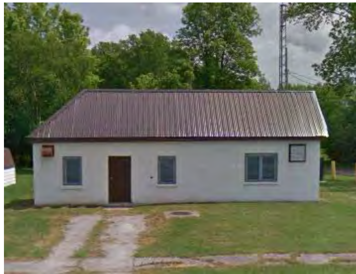
Figure 2 – Pumping Station No. 2
