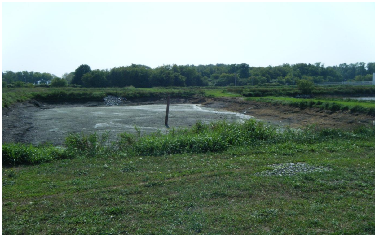
Photograph 2: Looking south at a wastewater treatment pond
