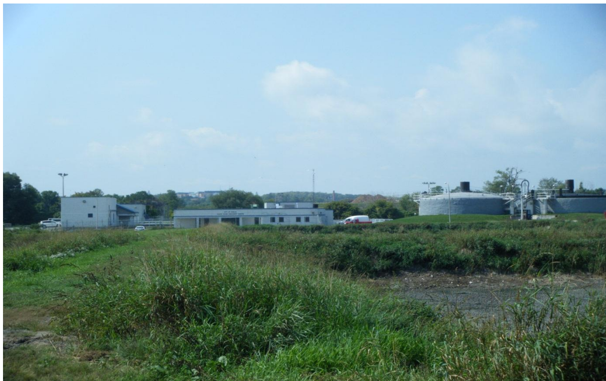
Photograph 1: View of Wastewater Treatment Centre looking southwest from the Snow Dump
