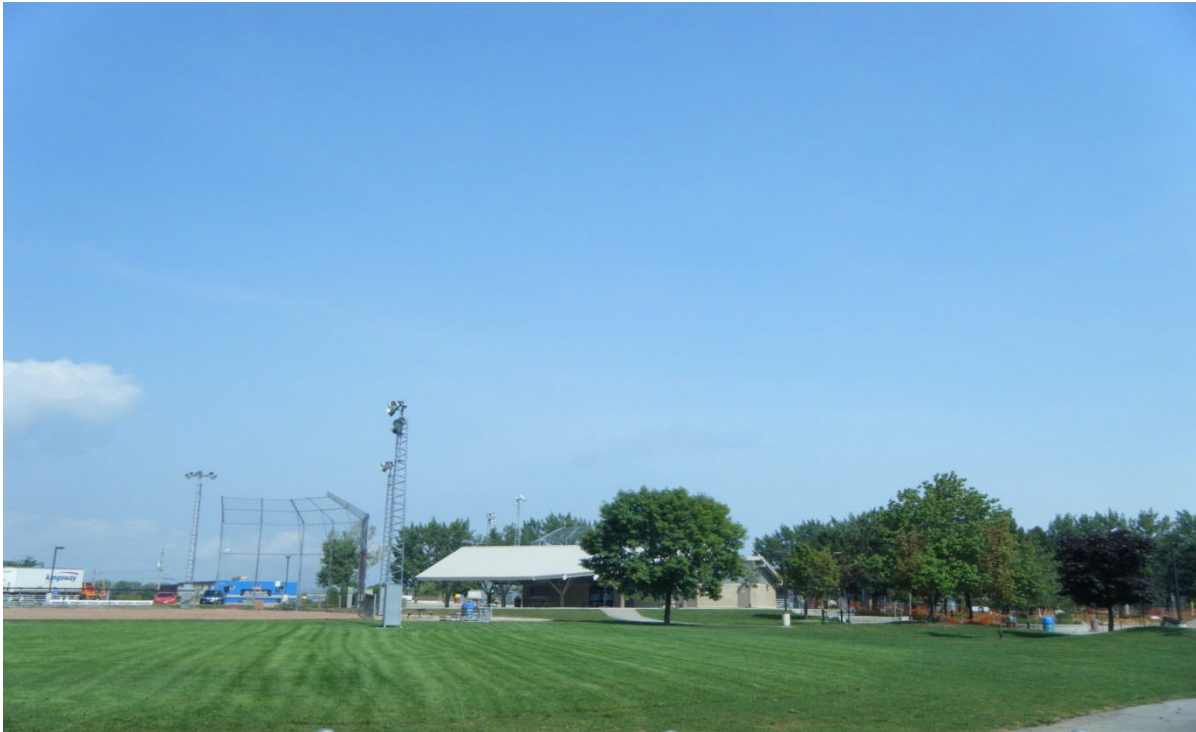
Photograph 3: View of the central fill area of the Site noting the newly constructed building
