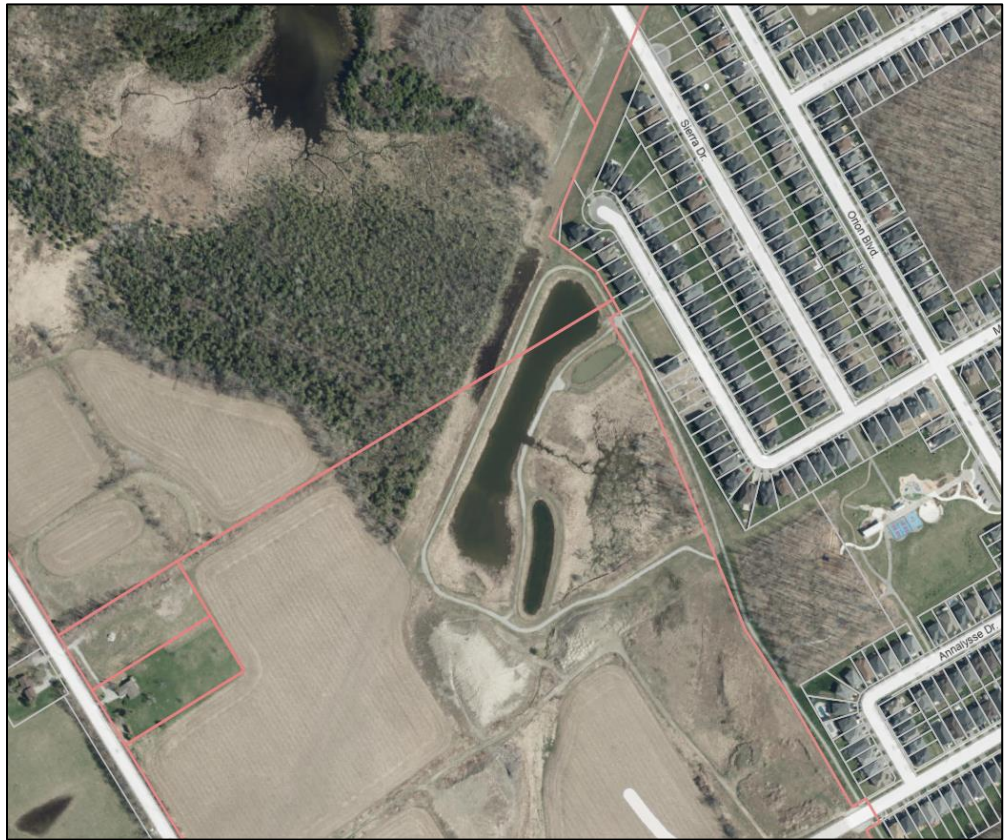
Figure 7 Simcoe County Aerial Photography 2025 of West Ridge Trailside
