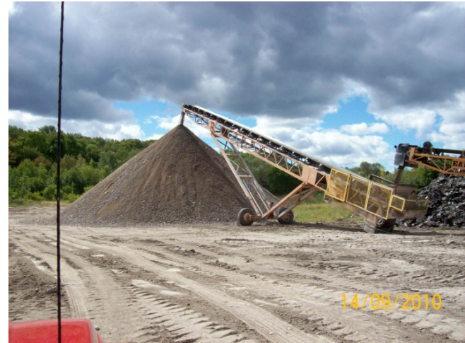
Crushed for reuse
