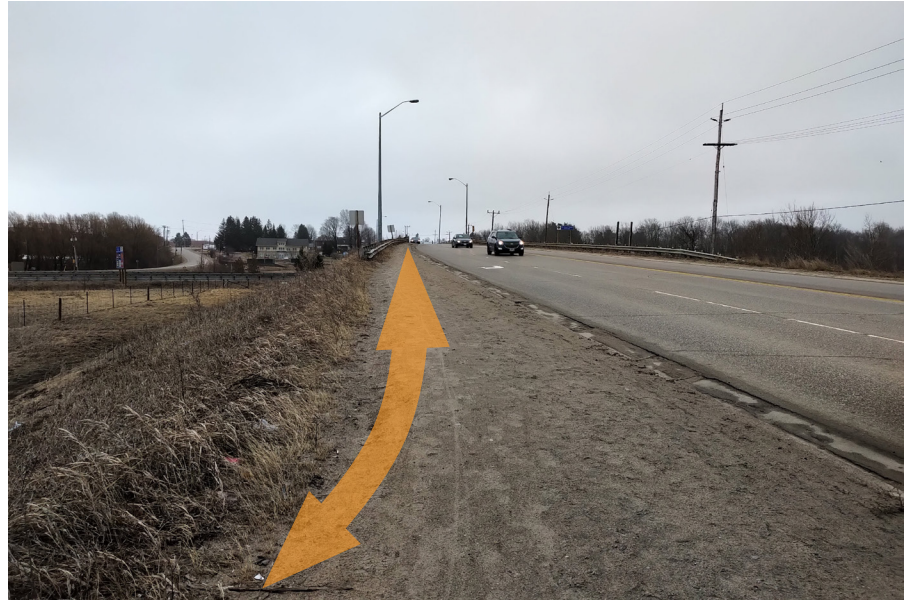
Figure 2.10 The existing West Street Overpass of Highway 11 has a grass desire line from all the pedestrians that use it to access the retail plaza north of the highway. There are currently no pedestrian facilities.
