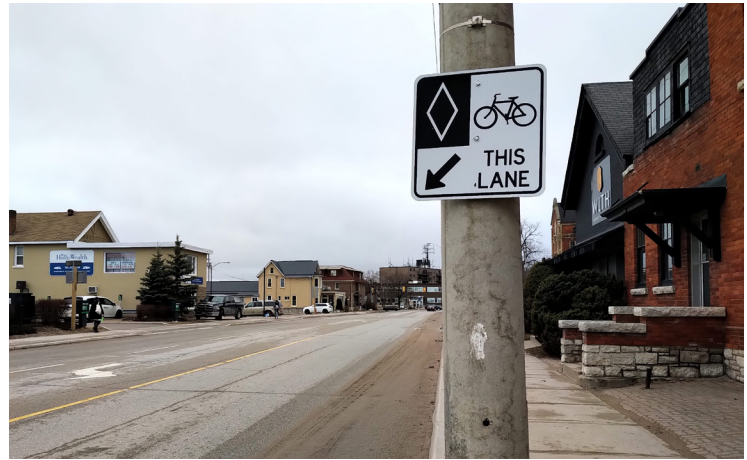
Figure 5.27 Example of the impact that winter sand has on bike lane markings on Coldwater Road
