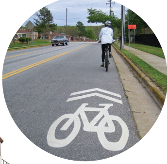
Figure 5.4 Typical cross-section with sharrows
