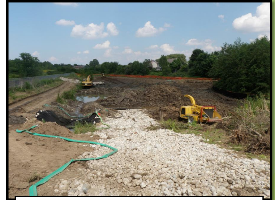
Construction of a Storm Pond
