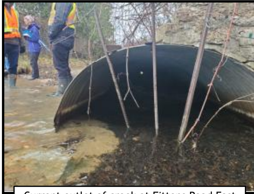
Current outlet of creek at Fittons Road East
