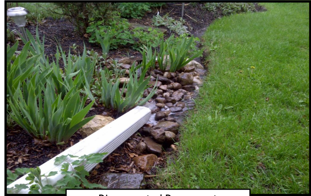
Disconnected Downspout
